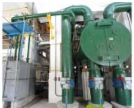
The design of this plant hinges around the idea of encapsulating all the wasted heat from the production system and using this steam to heat up boilers which eventually runs the turbine, thus producing electricity. The estimated annual CO<sub>2</sub> reduction by virtue of WHR Plant at Pezu is 29,918 metric tons and at Karachi plant it is 50,000 metric tons.
